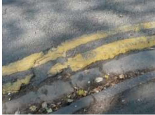
Photo 54: Evidence of cobbles under tarmac
