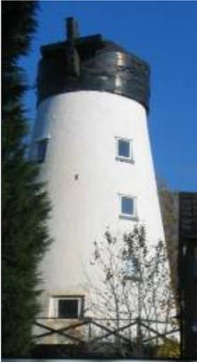
**Figure 43 Inappropriate windows in the windmill**
