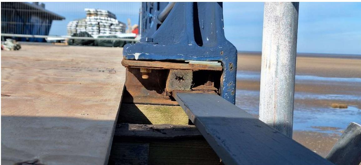
Photograph 74 – 2-Bolt Handrail base connection on North side of Area 1
